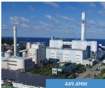
The Donghae Power Complex is a fluidized bed power plant that uses anthracite produced in Gangwon-do as a power generation fuel. It contributes to maintaining the local coal mining industry, and recently, it has initiated the operation of a biomass power plant that uses abundant local waste wood as fuel, thus building an ecosystem for the related industry.
