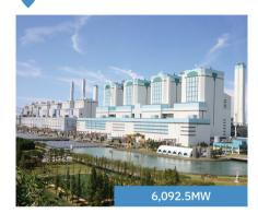
The Dangjin Power Complex serves as EWP's core power plant, playing a pivotal role in the power supply in the central region of Korea. It pursues pollutant minimization in the process of power generation, such as pollution control facility improvement projects, including the replacement of the flue-gas desulfurization (FGD), deNOx system, and adding indoor coal storage to reduce fugitive dust.
