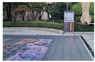
Application of "pavement block solar power"
